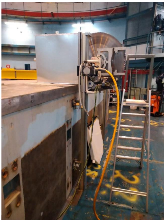
Figure 16: The saw was mounted and ready to make the first cut.
