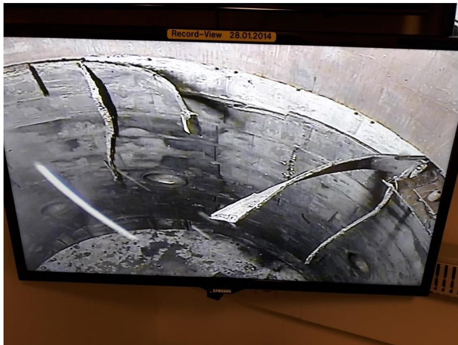
Figure 13: Lead sheets being peeled off
