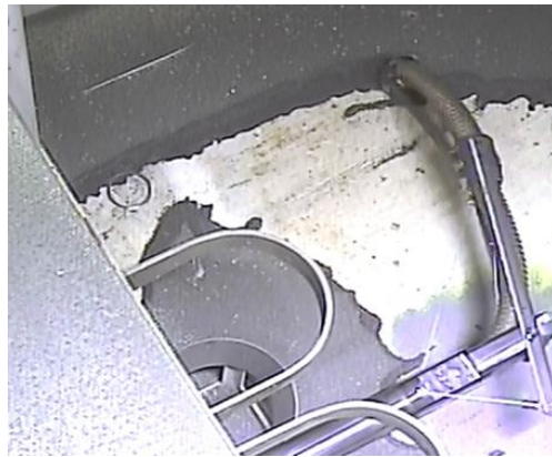
Figure 24: Remote vacuum cleaning in one of the Hot Cells
