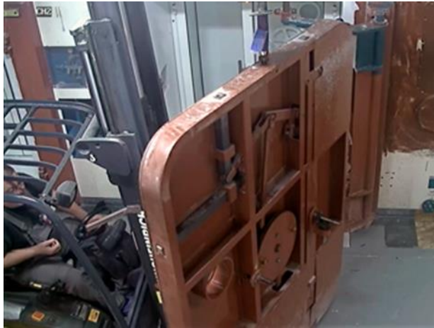
Figure 26: Outer “alpha” doors being removed from the back of the cells.
