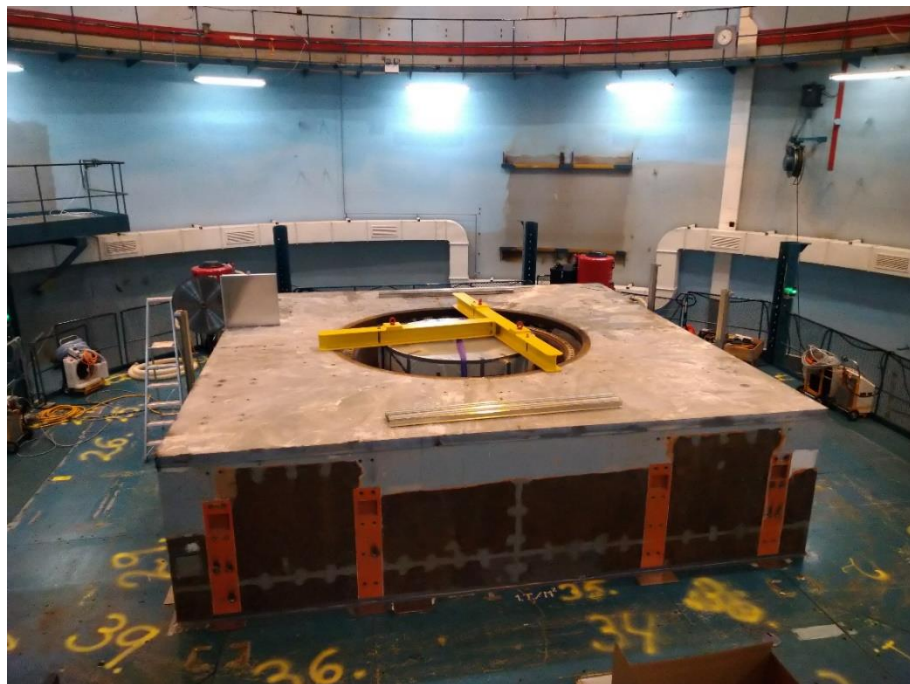
Figure 15: The deck around the biological shielding has been lowered.
