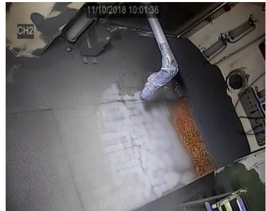
Figure 23: Sandblasting a table in Hot Cell no. 6
