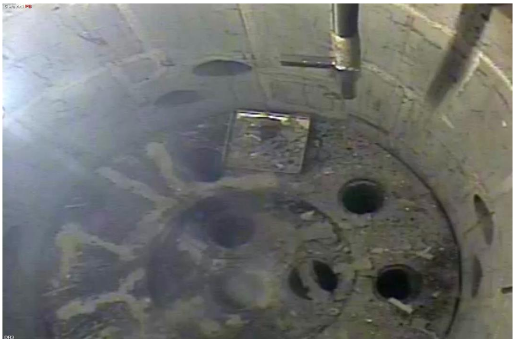
Figure 4: RAT has been cut up and taken out. Next step is vacuuming.
