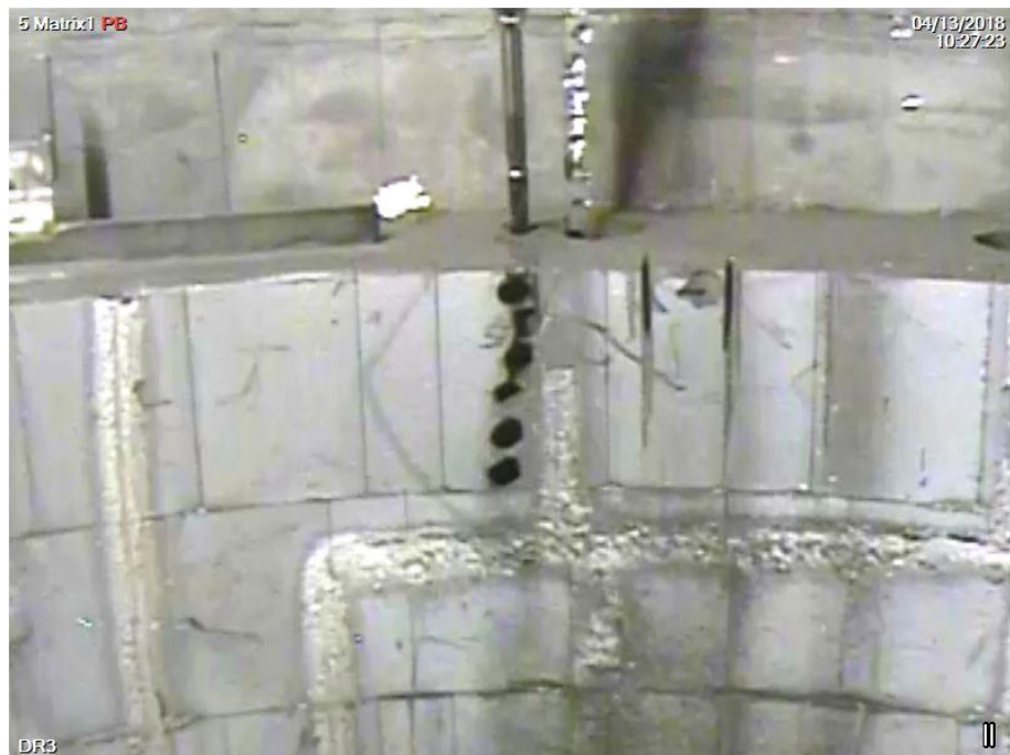
Figure 10: Vacuum lifter in use.
