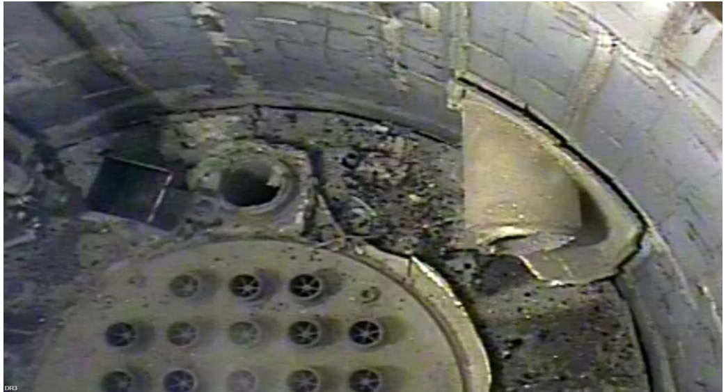
Figure 3: Inside the reactor, grid plate and experimental tubes
