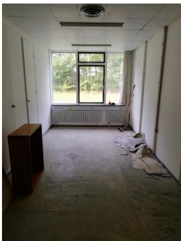
Figure 34: Non-active office area prepared for contamination survey
