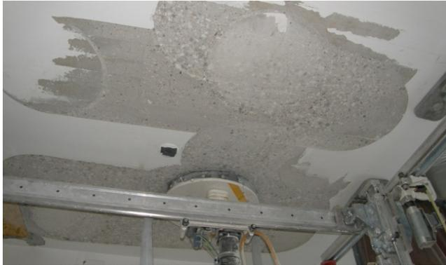
**Figure 30: Wall shaver during shaving the ceiling in the powder room**
