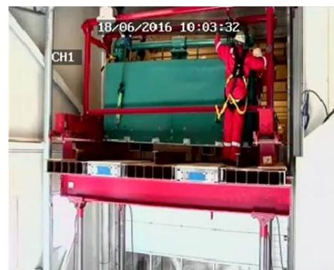
Figure 24: The last shutter house with shutter inside is being removed.
