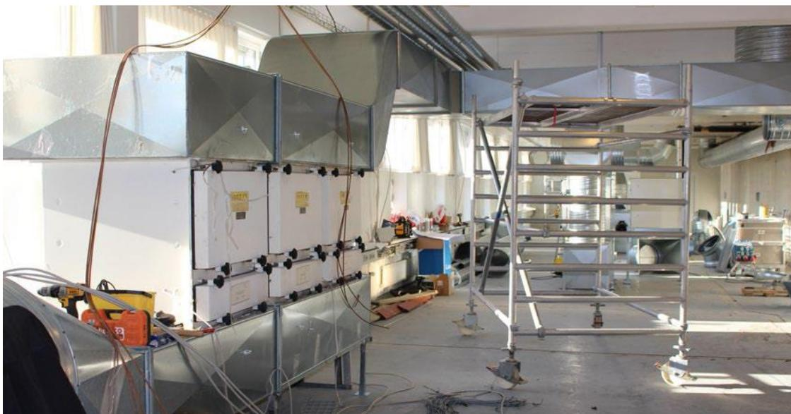
Figure 21 : Filters from the roof are now placed inside the facility
