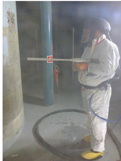
Figure 7: Removal of paint containing PCB with dry ice blasting on the ISB before scabbling
