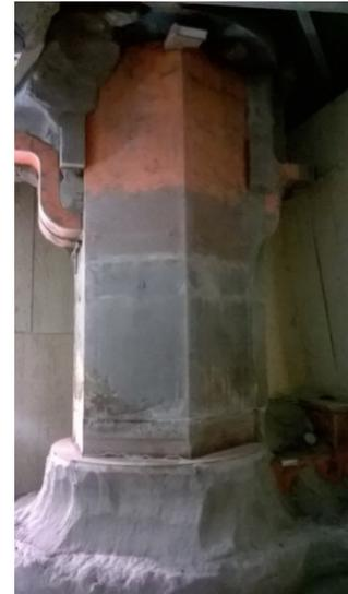
Figure 9: Shot concrete on the back side of the ISB.
