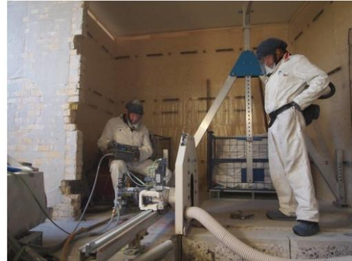
**Figure 31: Sawing of the floor in the powder room.**
