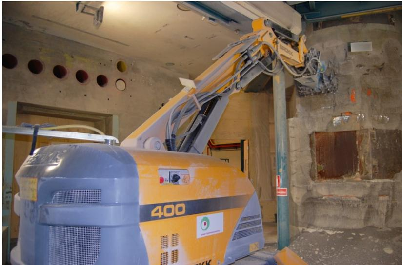
Figure 8: Removal of shot concrete from the ISB next to the D<sub>2</sub>O plant room by use of a scabblor on a Brokk.
